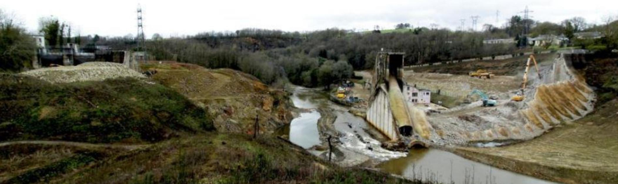
Vezins dam 13 january 2020 : 80 % of the 36 m high dam removed © DDTM50 in coop. with ERN
