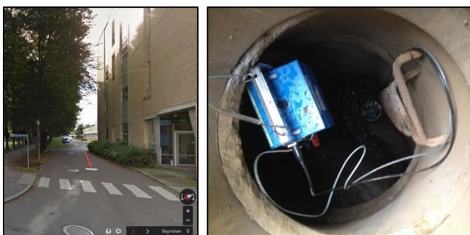
Figure 1. Automatic sampler and flowmeter mounted in manhole at Ullevål hospital.
