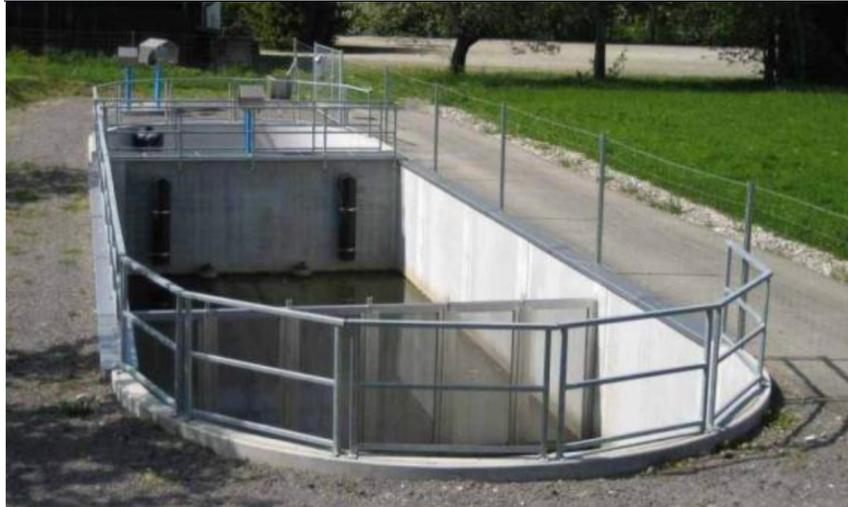
**Figure 6.18 Units based on filtration:** A pre-sedimentation catchbasin (in front) and a down-flow media filter treating first flush (15 min, one-year return period) in Austria (Photo: Courtesy of ASFINAG).
